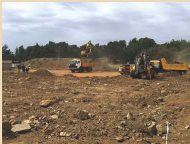
Ground preparations in full swing.
